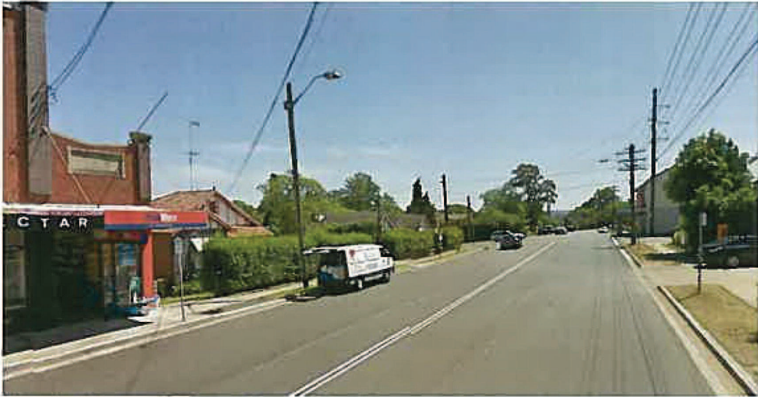
View looking north along Monash Road
